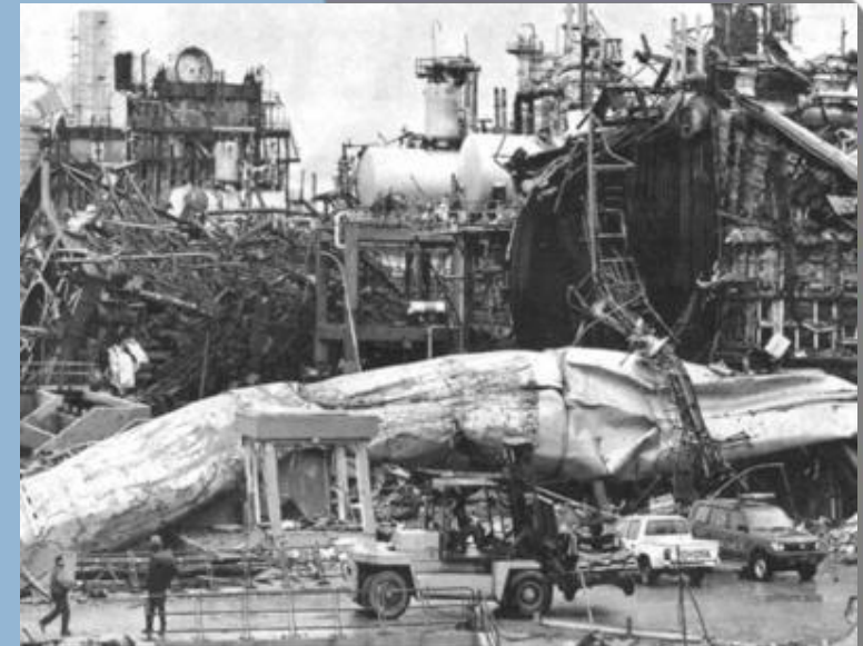
Skikda LNG plant, Algeria (2004) LME induced explosion in cold box 27 killed, 72 injured, cost US$30,000,000
